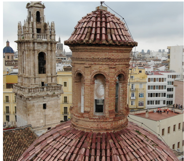
Figure 2: Detail view of the dome of the Santo Domingo Convent, Valencia for heritage inspection.
