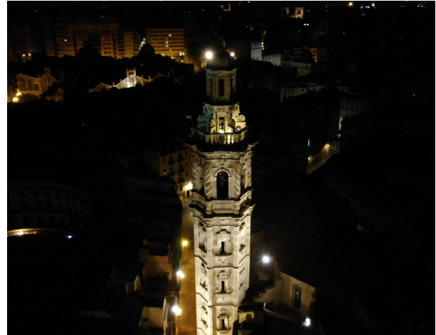
Figure 1: Public light inspection at Santa Catalina's Church, Valencia
