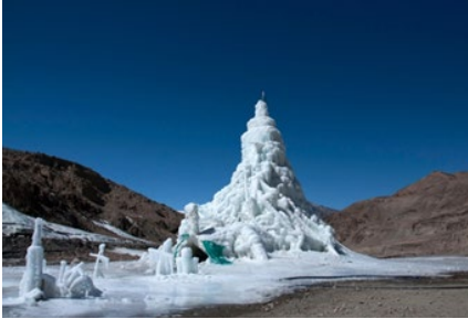
Figure 1. Ice Stupas create freestanding caches of water for irrigation, held in the winter as ice. Source: Carey Clouse
