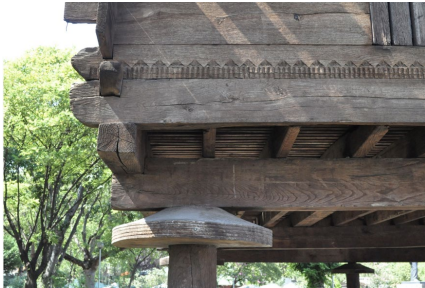
Figure 7. Tectonics in Serander detail of the corner & ornamentation, Trabzon, Turkey. Source: (Author 2014)
