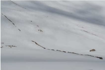
Figure 2. Snow Barrier Bands are built on mountain passes to catch and divert wind-blown snow for irrigation use. Source: Carey Clouse
