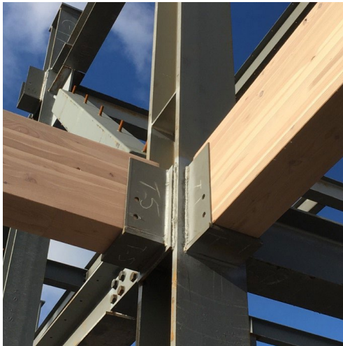
Figure 5.6. Carbon12 Detail, Beam - Steel Core Connection with adjusted glulams. Source: (Kaiser+Path n.d.)
