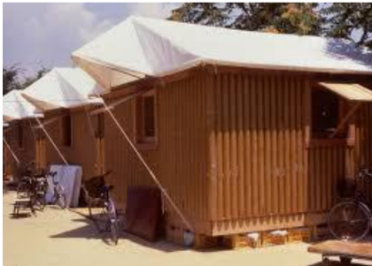
Figure 3. Paper-Log-House in Kobe
