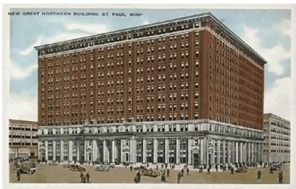
Figure 3. Railroad and Bank Building. Source: City of Saint Paul and the Saint Paul Heritage Preservation Commission (1988).
