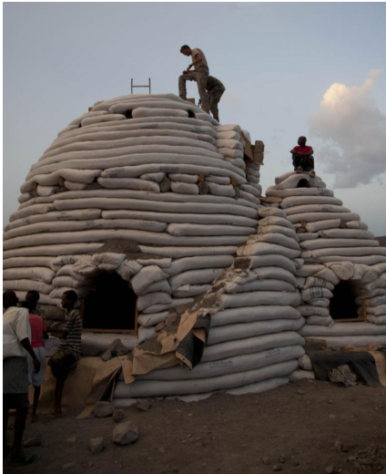
Figure 5. Figure 5: Superadobe sandbag shelters in Djibouti in 2012
