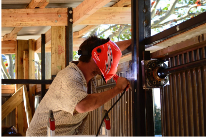
Figure 3. Constructing the mechanism for the rotating walls using scavenged bearings (Shall 2019).
