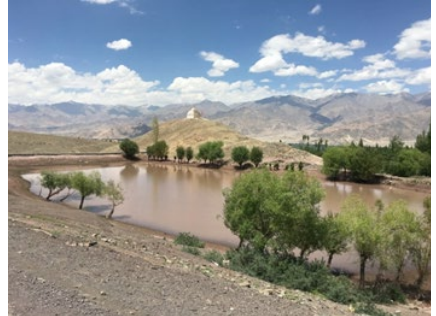
Figure 4. Water reservoirs are built into the landscapes above village farms and below glaciers, to hold irrigation water for equitable shared use, as a form of the commons. Source: Carey Clouse
