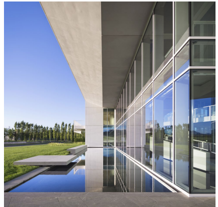
Figure 2. Italcementi i.lab in Bergamo, by Richard Meier.
