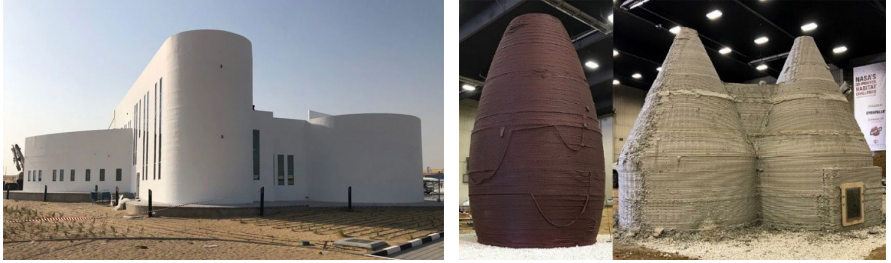
Figure 4. Examples of 3D-printed construction; office building in Dubai (left); constructions in NASA contest (right). Sources: ( https://www.apis-cor.com/ , https://spectrum.ieee.org/tech-talk/aerospace/space-flight/3d-printers-could-build-future-homes-on-mars , photographer Tracy Staedter)
