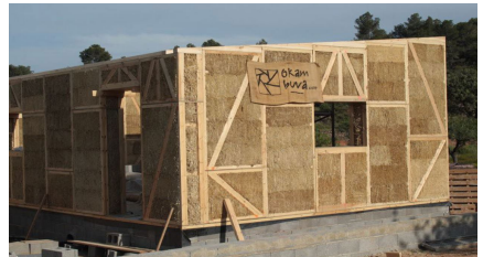
Figure 1. Construction process using rice straw panels.
