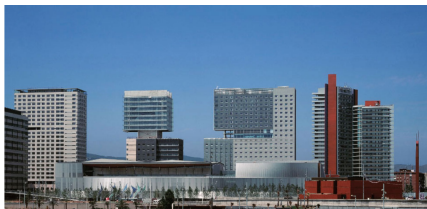
Figure 1. Forum 2004 area. Photographer Duccio Malagamba
