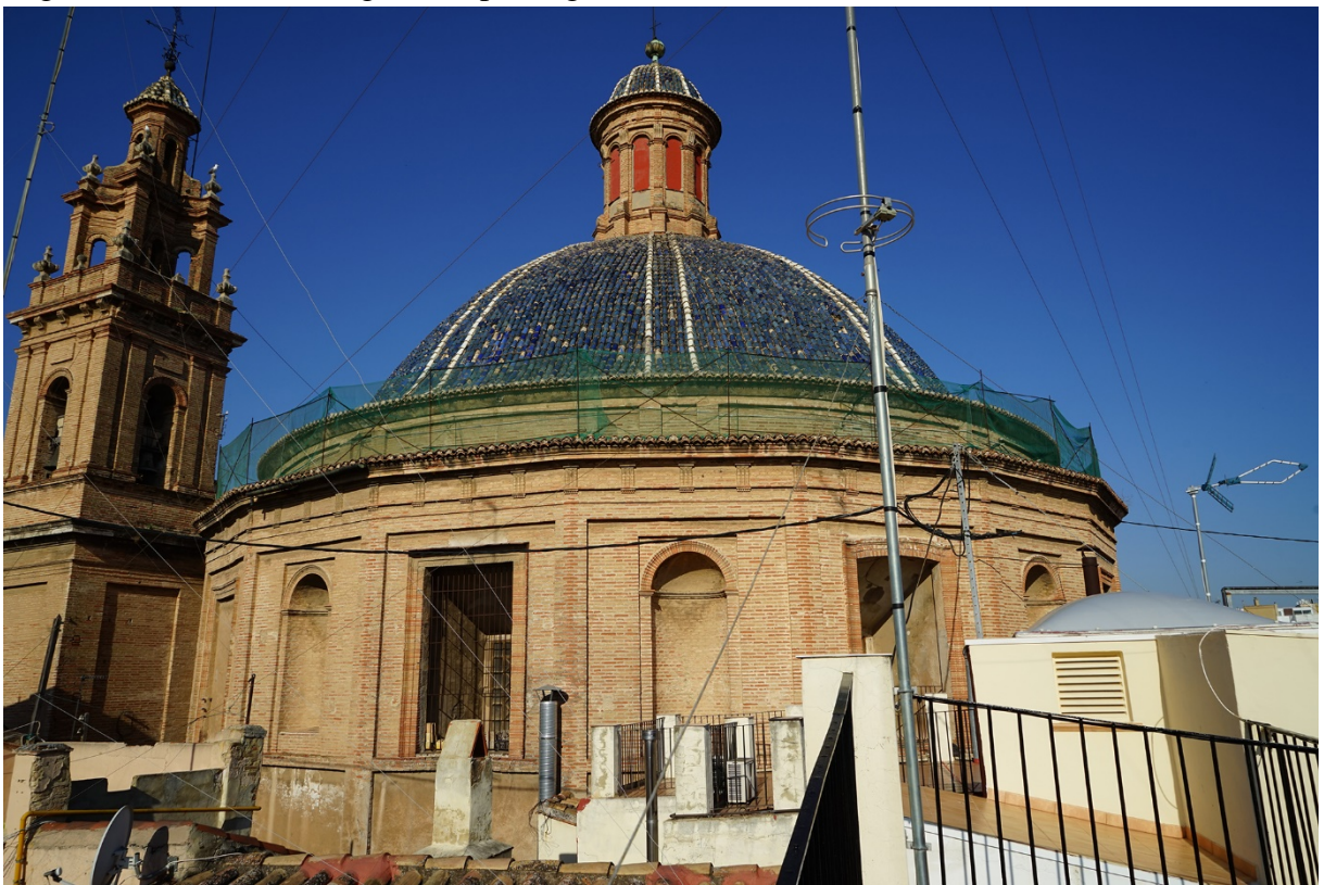
Fig. 6 Exterior of the dome where splayed openings and outside niches can be observed. Source: Rodríguez-Navarro & Gil-Piqueras
