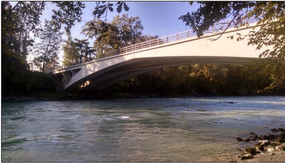
Fig. 13: R. Maillart's Vessy bridge (1937) over the Arve River in Geneva, Switzerland. The underside of the arch is not a continuously smooth curve from abutment side to abutment side like in Salginatobel, which enabled Maillart to express visually the discontinuity created by the hinge at the crown. Image: M. Garlock.
