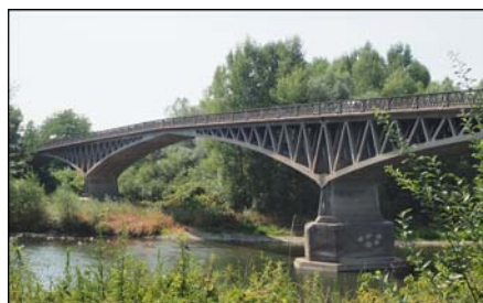
Fig. 8: E. Freyssinet’s Boutiron Bridge (1912) over the Allier River in Creuzier-le-Vieux—Charmeil, France. Image: I. Paya-Zaforteza
