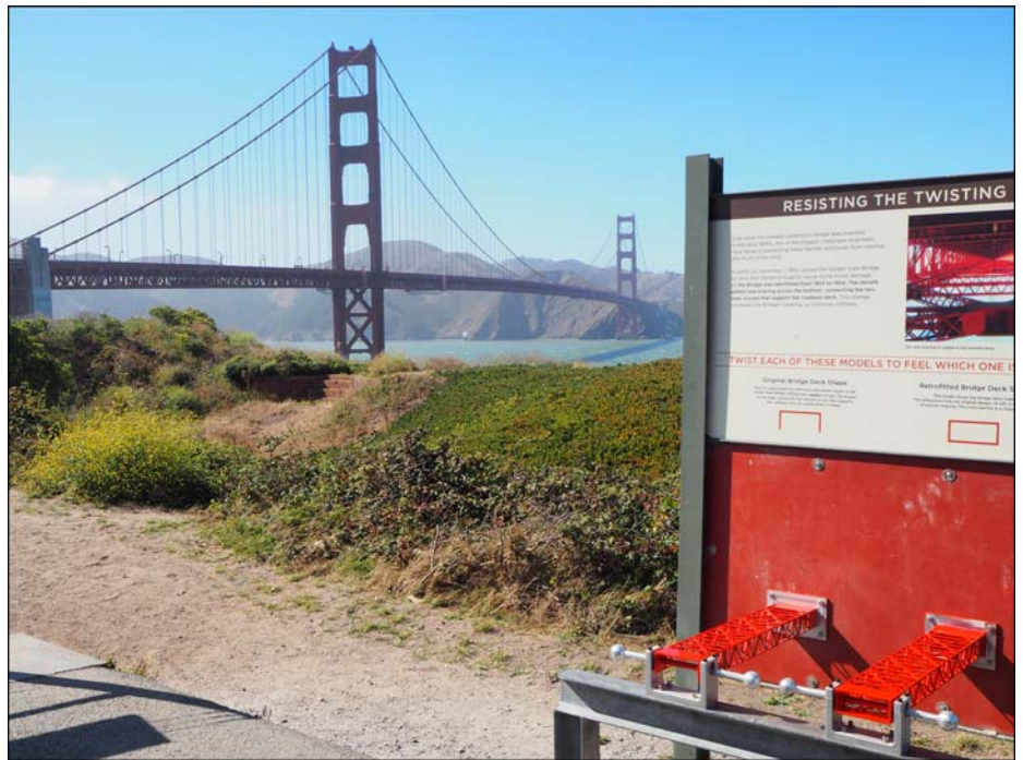
Fig. 7: Golden Gate Bridge. General view and explicative panel at the Golden Gate Bridge exhibition showing two scale models of a portion of the bridge deck. The one on the left is the original open section. The one on the right is the retrofitted section. Image: I. Paya-Zaforteza
