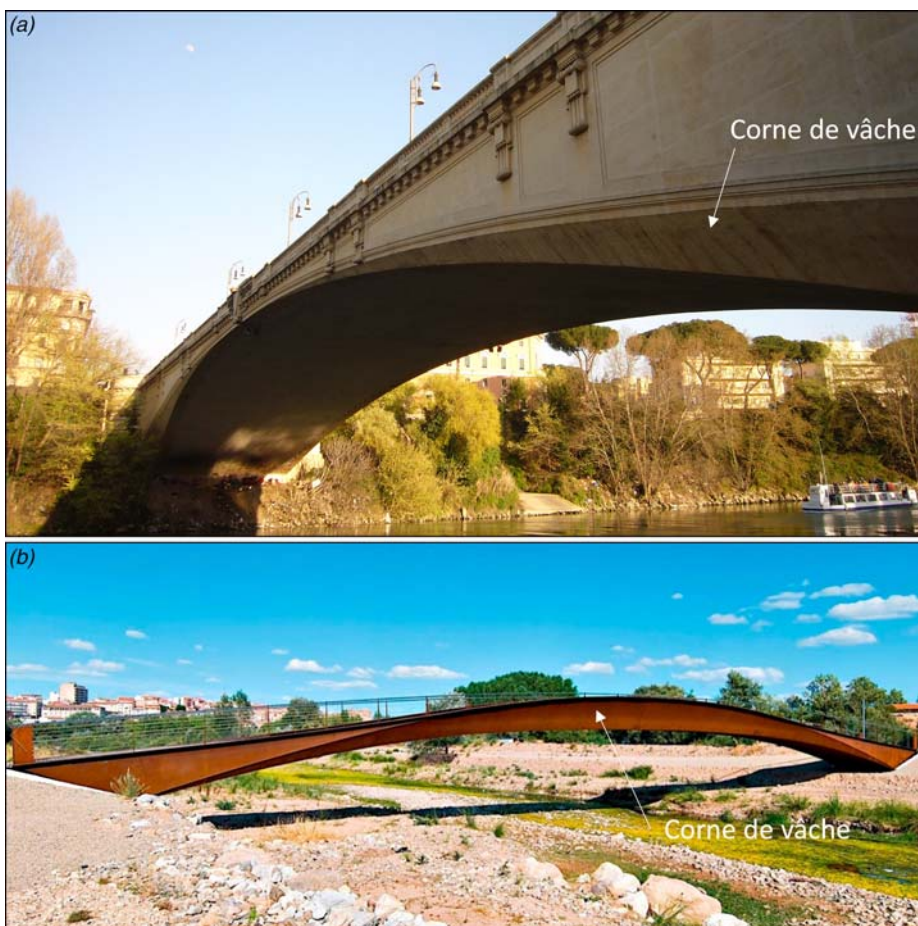
Fig. 4: (a) F. Hennebique’s Resorgimento Bridge (1911) over the Tiber River in Rome, Italy. Image: I. Paya-Zaforteza. (b) M. Guisasola’s Calahorra Footbridge (2007) over the Cidacos River in La Rioja, Spain. Image: José Manuel Cutillas (courtesy of Anta Ingeniería Civil)
