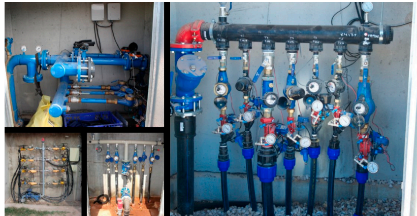
Figure 2. Variable configurations of multioutlet hydrants in the field.
