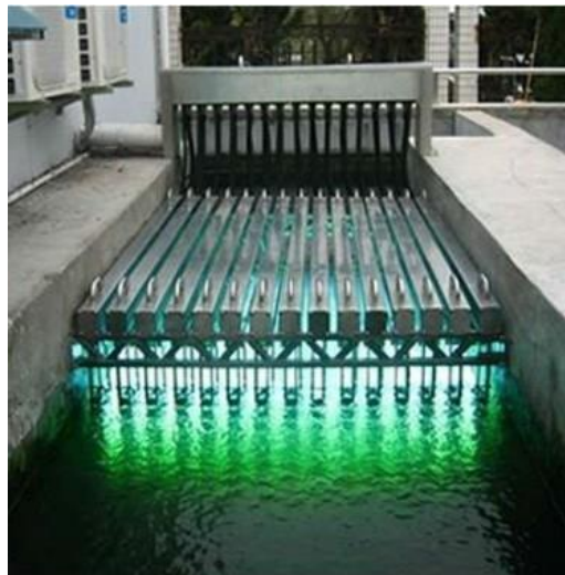
Figure 1.16. Water treatment by UV-C radiation.
