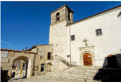
Fig. 4. The church of S.Maria Assunta before the earthquake of 2016 (Source: http://www.sabap-umbria.beniculturali.it/index.php?it/257/norcia-fraz-castelluccio ).
