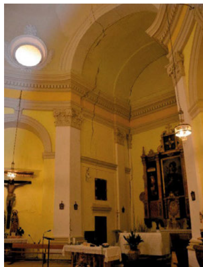
Fig. 4. Interior view of the church (Source: The authors, February 2022).
