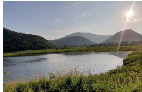
Fig. 2. Sareed Phong Earth Dam (Source: Pittungna-poo, 2020).
