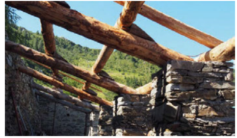
Fig. 4. Construction site in “Baita Eterna” ( https://fondoambiente.it/ ).
