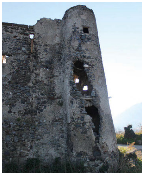
Fig. 8. Fortified house Casillo. Detail of the tower on the southern side. The wall structure is also visible here, with irregular stone elements of different shapes and the use of abundant mortar (Source: Ragosta, 2022).
