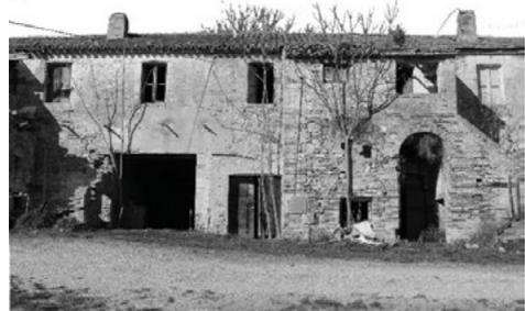
Fig. 7. Transformations of farmhouses. The construction of extension followed height and volume of the origin building, emphasizing the longitudinality of the façade. (Source: Cipolletti & Guaiani, 2022).
