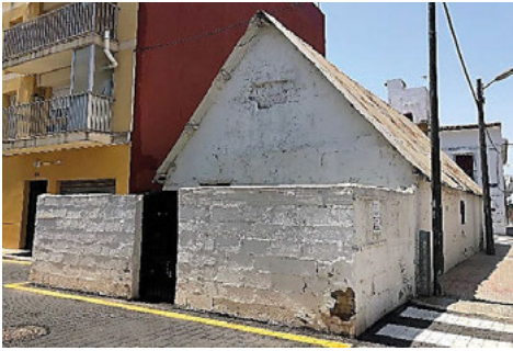
Fig. 7. Isolated Valencian barraca , in a district of Valencia. This traditional local architecture is made of adobes, and it was once primarily spread around the city's territory. Today only a few examples have endured, and most of them are surrounded by the presence of modern buildings which have no connection with the traditional architecture and urban morphology (Source: Caruso, 2018).
