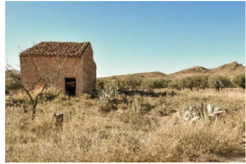
Fig. 8. Rammed earth abandoned building in Chodes, Aragón Community (Source: Caruso, 2021).
