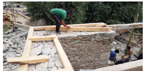
Fig. 18. Insertion of wooden tie beams ( sket shing ).
