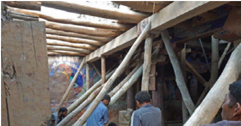
Fig. 12. Temporary beam at the entrance of the chamber.
