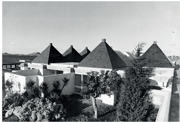
Figure 12. The Rubio house (La Manga). Defensive habitat/wall-enclosed patios.
