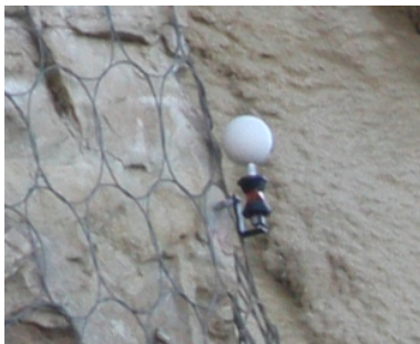
Figure 3. ChPs on the slope.
