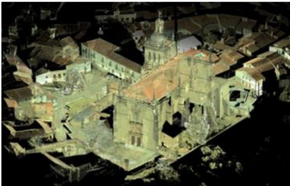
Figure 2. Full point cloud from the southwest view of Coria Cathedral.
