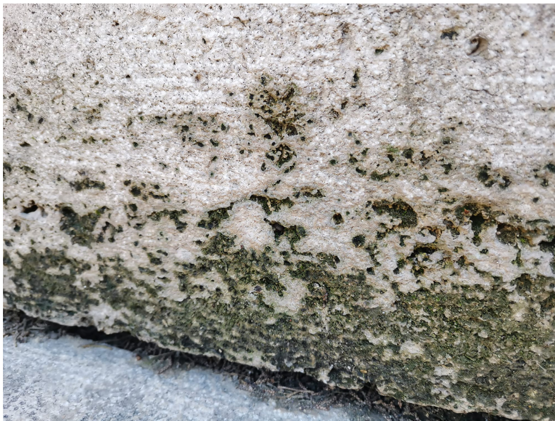
Figure 3. The cavities in the calcareous surface of artificial rock serve as an ideal space for growth of bacteria, fungi, and as depicted in the image, mosses
