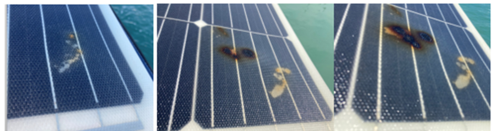
Figure 20. Development of hot-spots after three days of continuous use.
