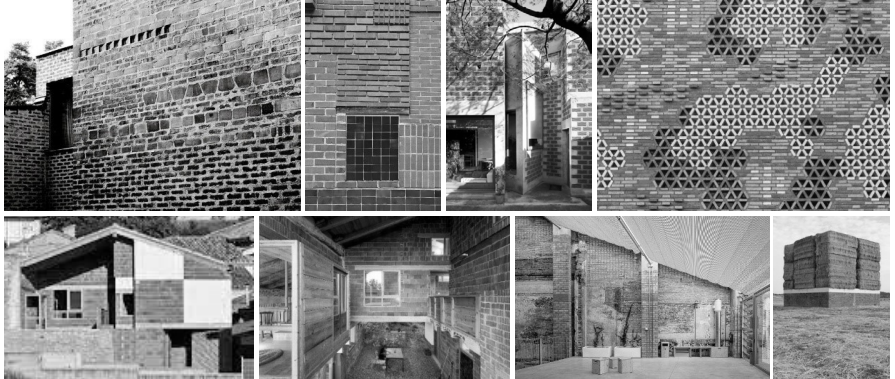
Figure 2. Comparative assembly of some of the examples given: 1- Lewerentz in Klippan; 2- Aalto in Muuratsalo; 3-Miralles in La Clota; 4- Benedetta in San Pau; 5 and 6-D. Sebastian in Three Springs; 7- Lleialtat Santseca Civic Center of the Harquitectes group; 8- Modulab at Harvest Moon Pavillion
