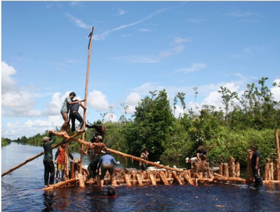
Peatland restoration blocking drainage channel. Wetlands International
