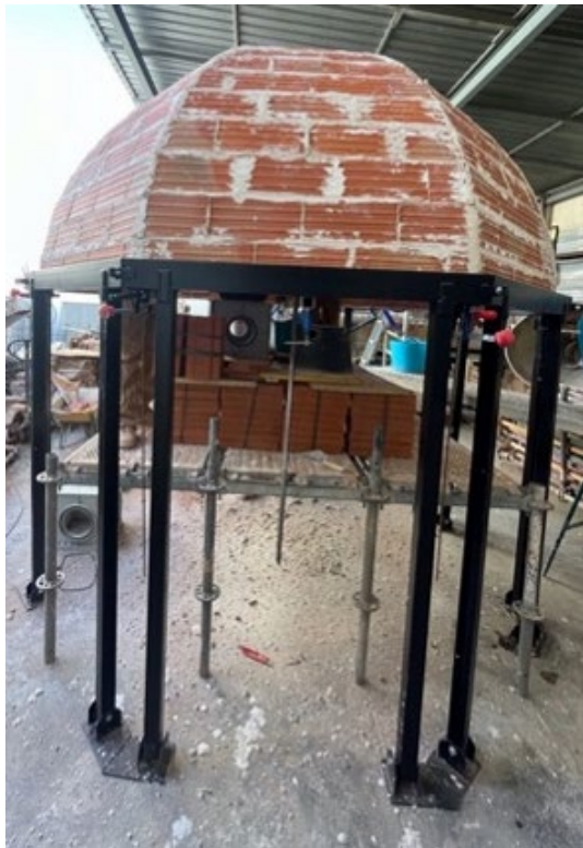
Fig. 8 - Real model built to test settlement cracks.
