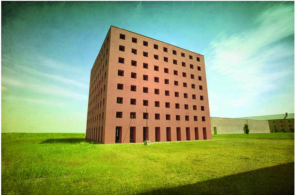
Fig 3. San Cataldo Cemetery, Aldo Rossi, Modena (Italy), 1971-1984. Photo by username-guiba6 in: http://www.plataformaarquitectura.cl/2011/02/01/clasicos-de-la-arquitectura-cementerio-de-san-cataldo-aldo-rossi/1292007831-sancat1/ 225x150mm (72 x 72 DPI)
