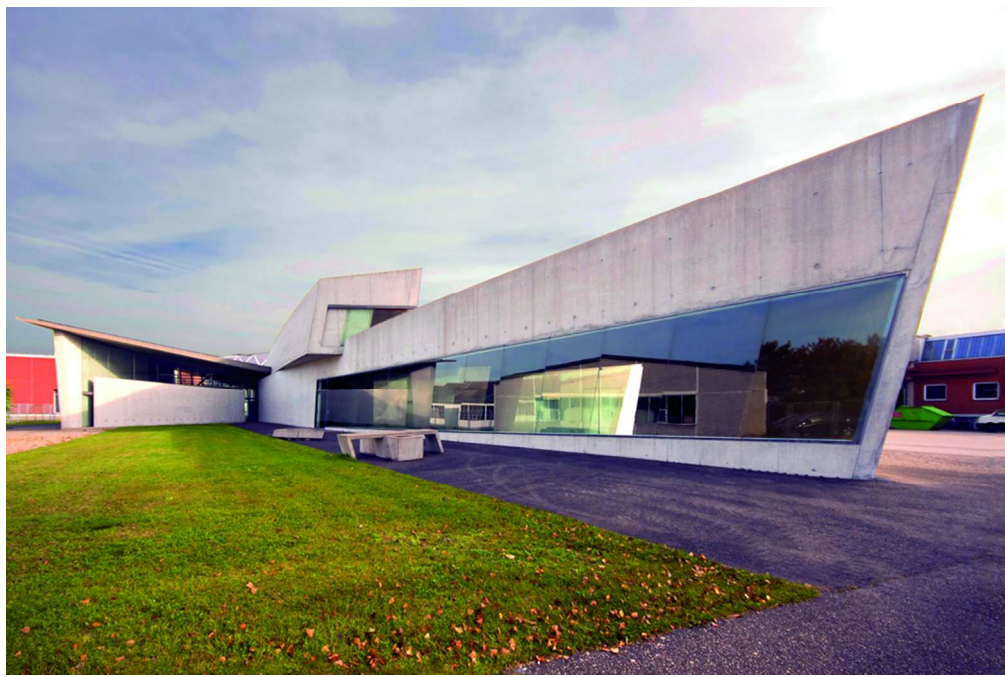
Fig 7. Fire station for Vitra factory, Zaha Hadid, Weil am Rhein (Germany), 1993. Photo by Wojtek Gurak in: http://www.flickr.com/photos/wojtekgurak/4121827372/ 352x235mm (72 x 72 DPI)
