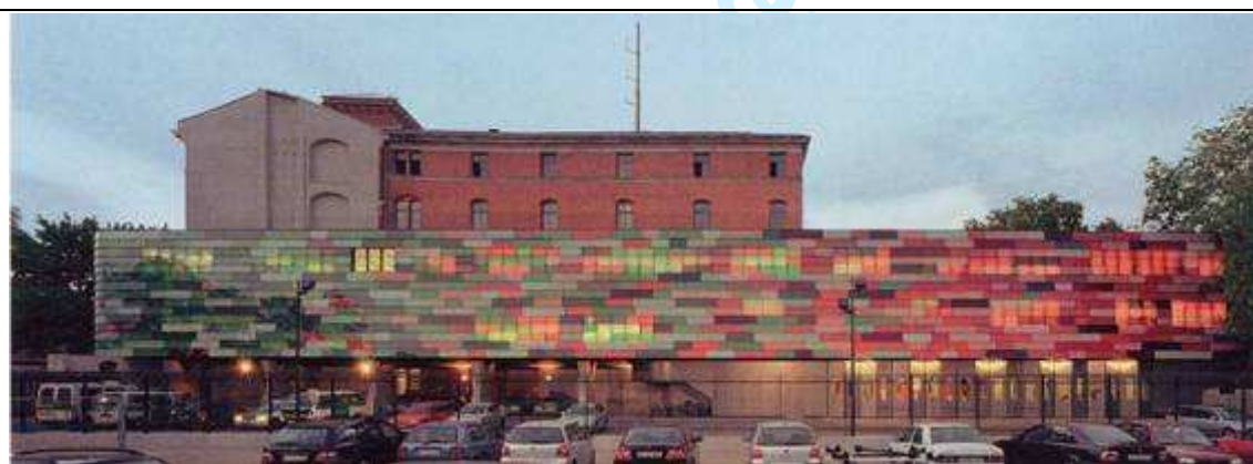
51 Fig. 37. Fire and Police station, Sauerbruch & Hutton, Berlin, 1999/ 2004. Courtesy Stucio Sauerbruch & Hutton 52 < http://www.sauerbruchhutton.de/ > 53 54 55 56 57 58 59 60
