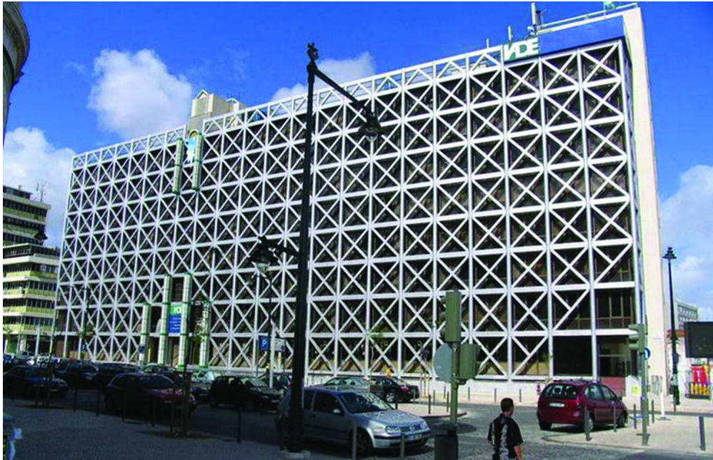
Fig. 20. Totovola Building (IADE), Tomás Taveira, Lisbon (Portugal), 1973-1984. 127x81mm (300 x 300 DPI)
