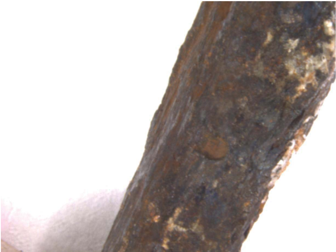
Fig.6. Joist wire with pitting corrosion
