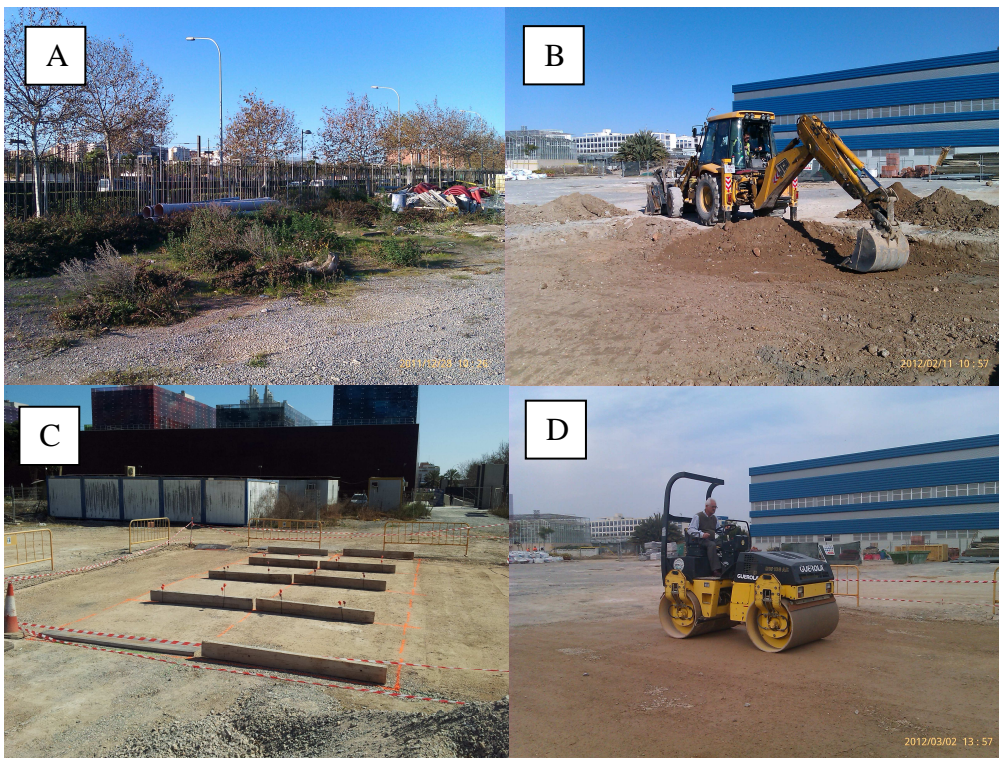
Fig. 3: Experimental platform construction process. A) Site before cleaning and clearing. B) Excavation. C) Site survey. D) Placing and compaction.
