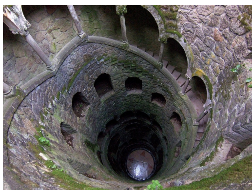
Fig. 125. The well in the form of an inverted tower in the Quinta da Regaleira
