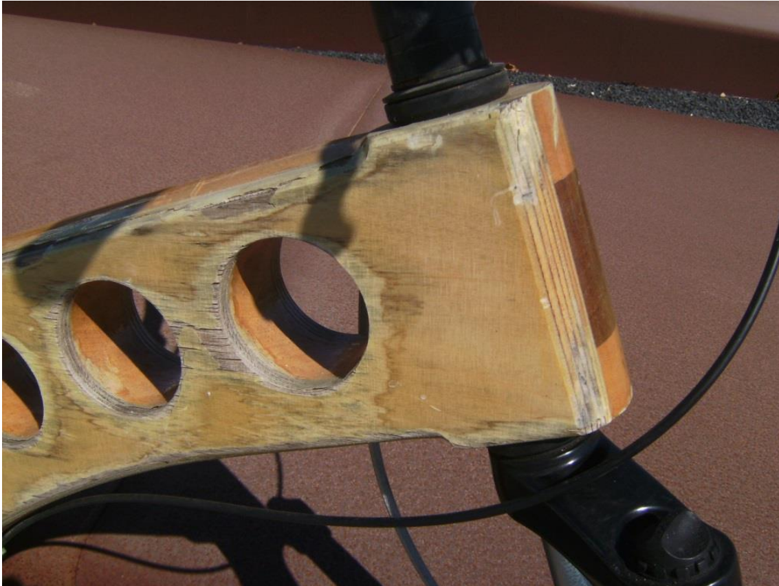
Figure 176. Lifting: In areas of water ingress lifting of the lacquer has occurred after prolonged exposure (5 years). Taylor, Nicholas. 2015
