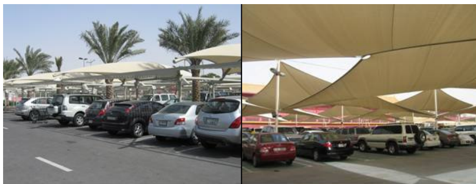
Photo 1: Mesh membrane structures
