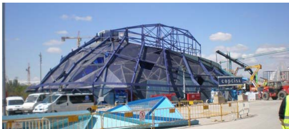
Figure 17. Additional structure between layers.
