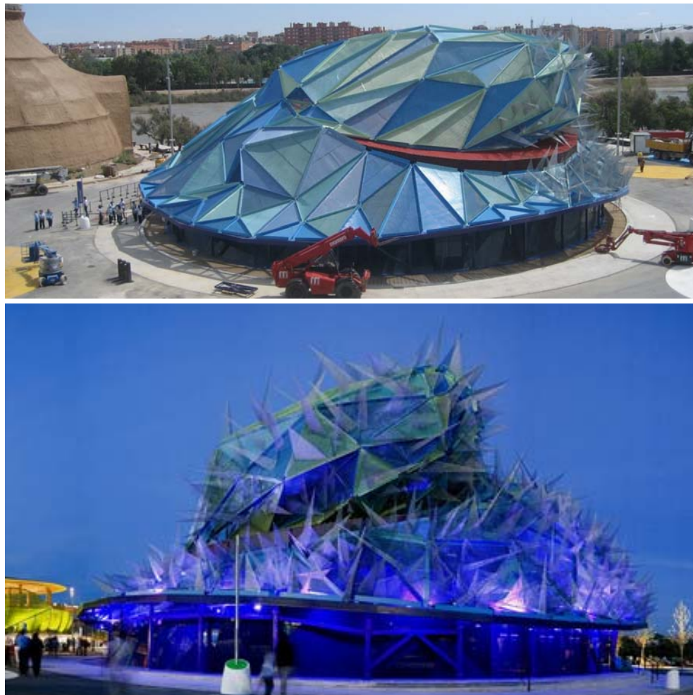
Figure 19. General aspect of the exterior of the finished pavilion.
