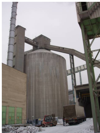
Figure 1: View of Clinker Silo PC2 with Technology
