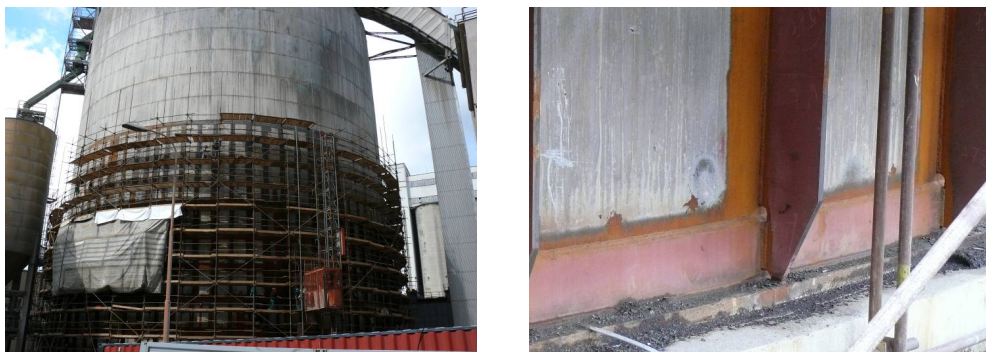
Figure 5: Reconstruction Works on the Clinker Silo
