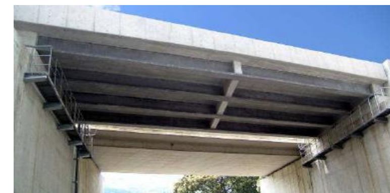
Figura 6 Puente Horikoshi C-Ramp [Tanaka et al. 2009]
