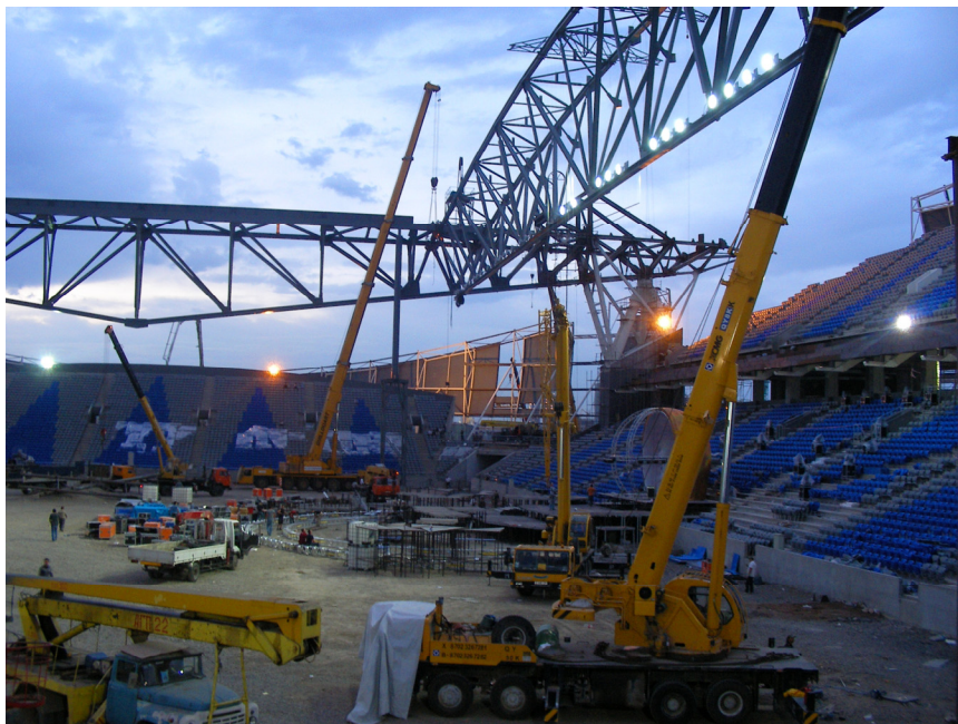
Figure 5: Erection of main roof trusses
