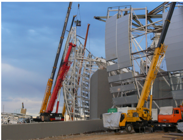
Figure 11: Side Wall Erection
