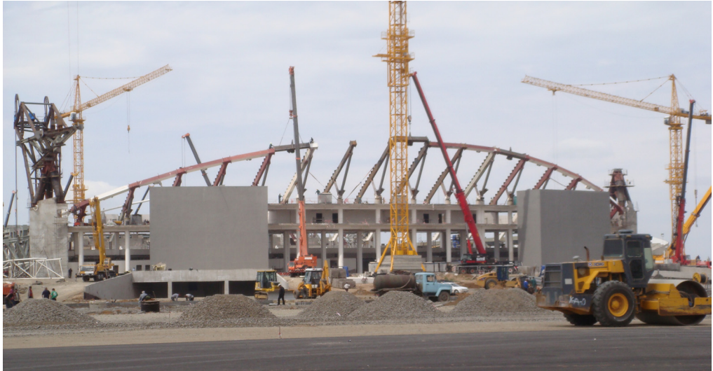
Figure 8: Tribune steel structure erection
