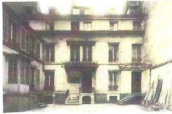
photograph before start of construction
