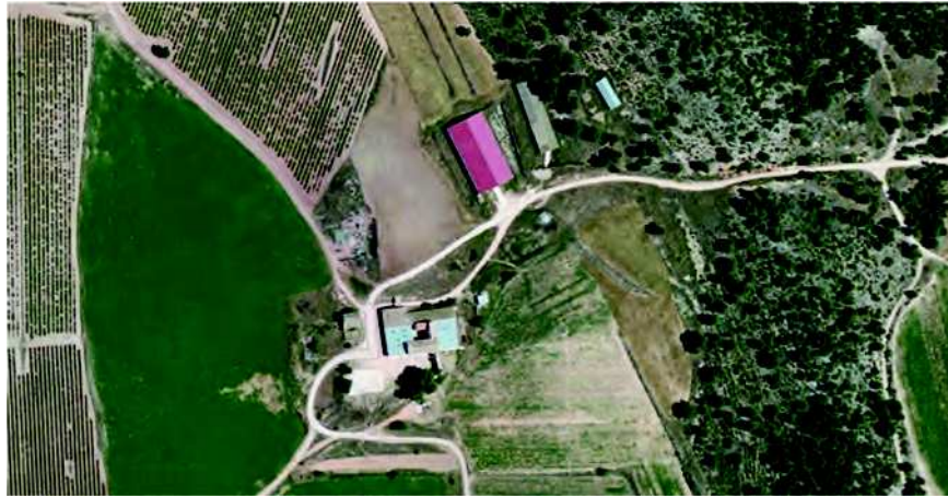
Figure 2: Industrial unit installation for a wine cellar, through a statement of community Interest in rural land, township of Ayora (Valencia).
