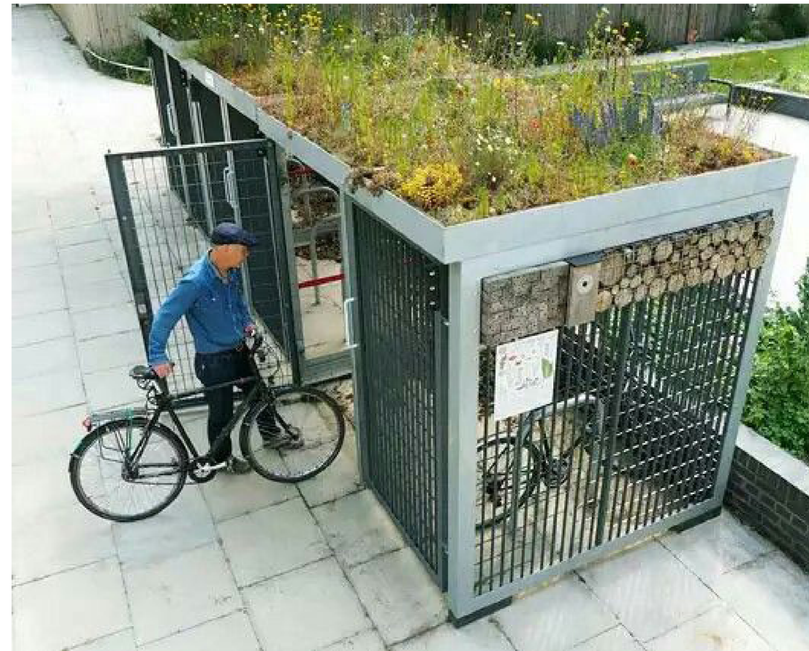
Fig. 66. Green roof bike shed. Reino Unido.
