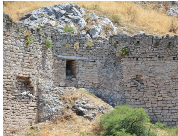
Figure 6: South elbow tower traces of lateral walls.
