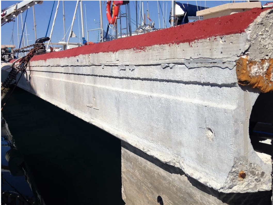
Figure 7.7: Photo of the prestressed, prefabricated slab of the pontoon
