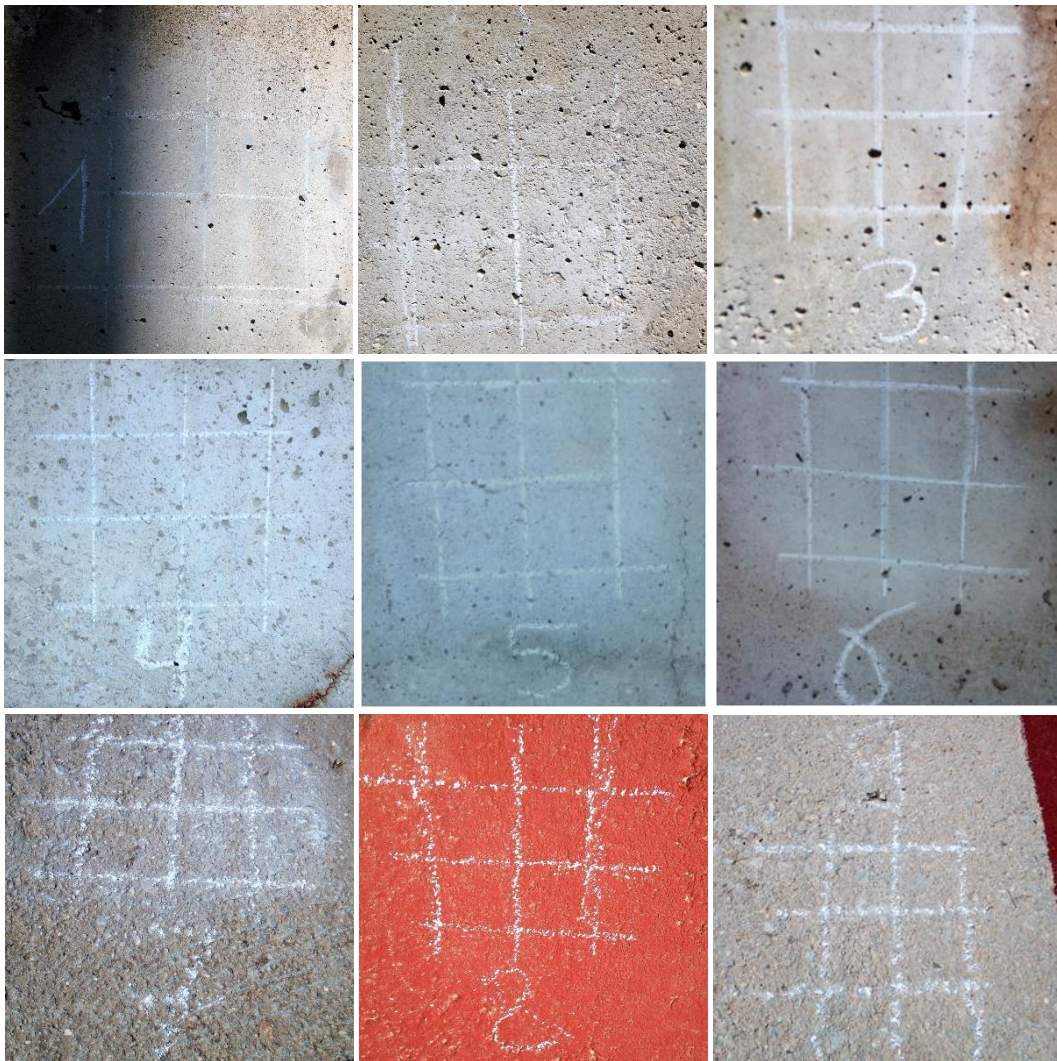
Figure 7.11: Photos of all the prepared areas for the rebound hammer test
