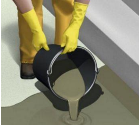
Figure 6.3: Pouring application of the repair mortar with formwork
