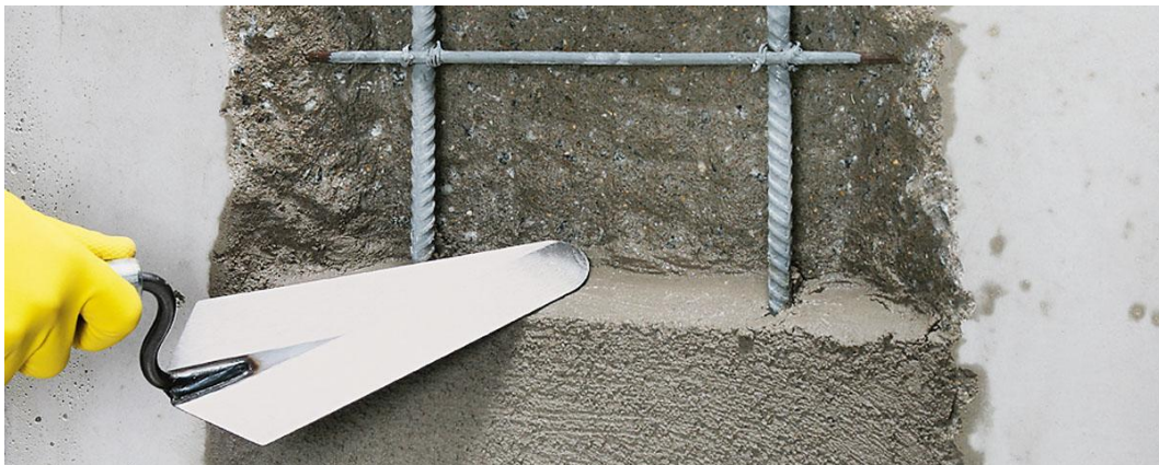
Figure 6.2: Manual application of the repair mortar with a trowel
