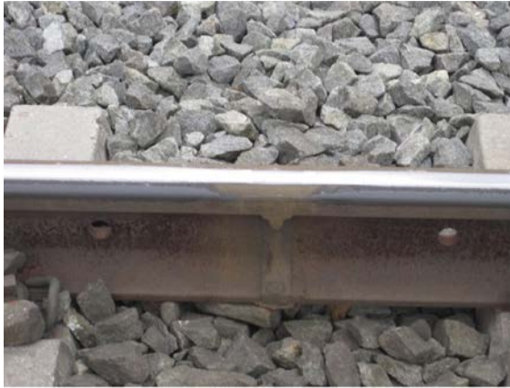
Fig. 5. Welded joint
