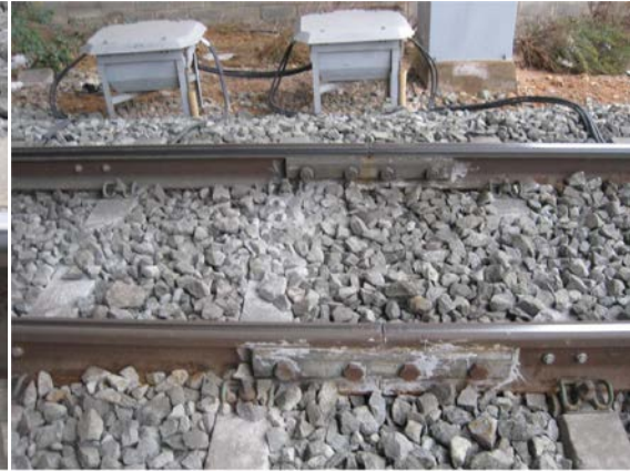
Fig. 6. Glued joint
