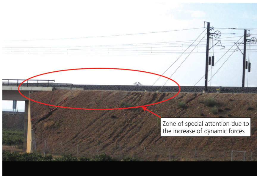
Figure 1. (a) Schematic profile of an embankment–bridge transition zone proposed by Adif. HS, hydraulic soil; GS, granular soil; E, embankment; B ballast layer; SB, sub-ballast layer; CF, form layer. (b) Transition zone built between an embankment and a bridge in the Madrid–Valencia high-speed line
