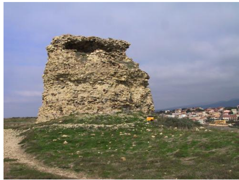
Fig. 2- Torre del Pozzo before the restoration
