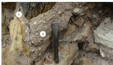
Fig. 11 – Detail of masonry with original (1) and repair mortars (2)
