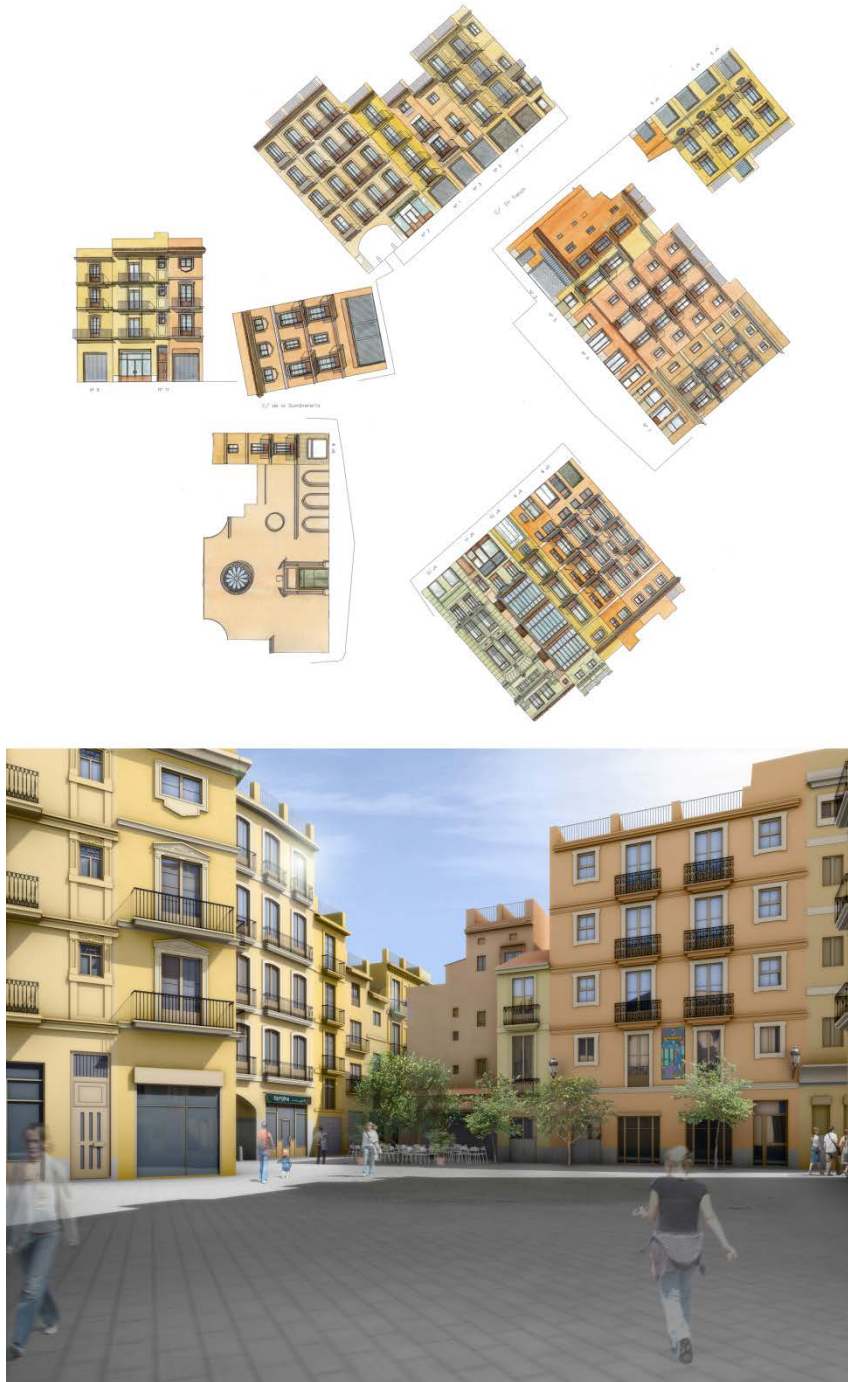
Fig. 7. Lope de Vega square. : An example of urban space with predominantly Artisan Buildings .
