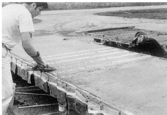
Fig. 2-18. Glass tubes in a bridge deck (Dry, 2000).
