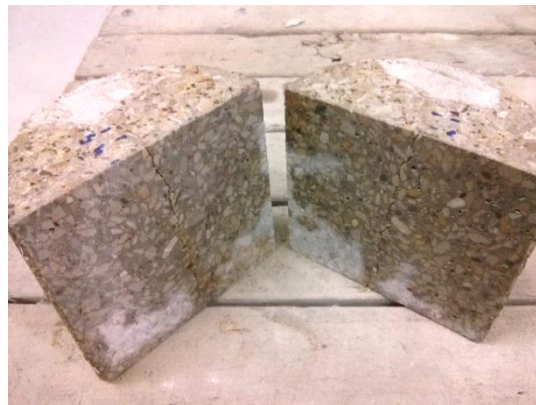
Fig. 4-20. Specimen with a transversal cut showing no precipitates in the internal part of the crack.
