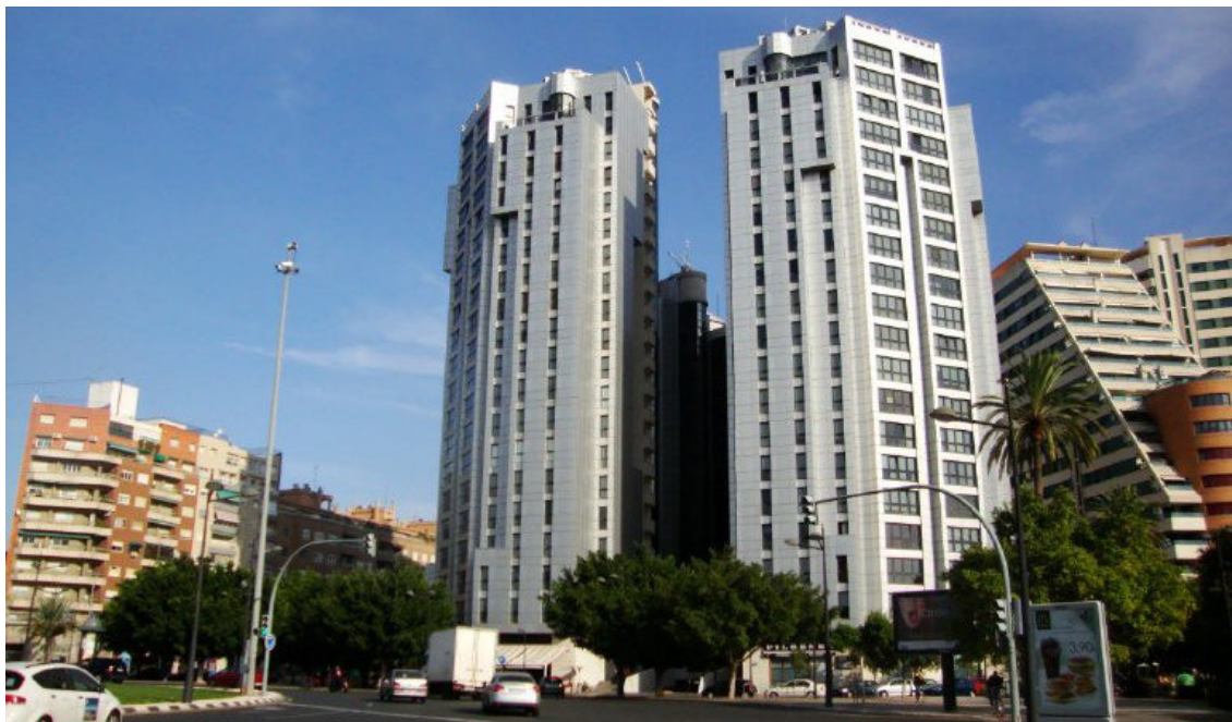
Fachada de Alameda House 38.
