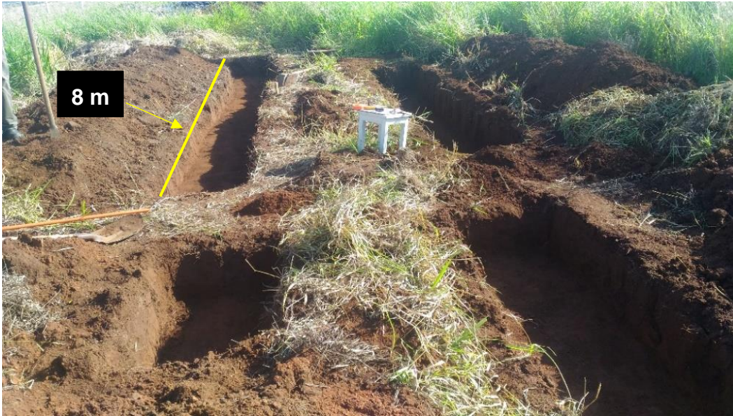
Fig. 3.4 Excavation of the ditches
