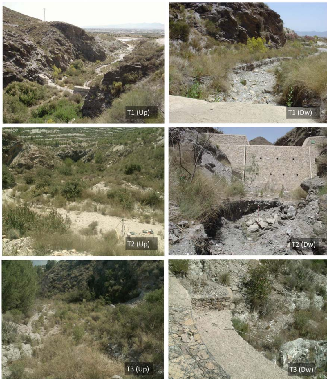
Figure 2. Riparian vegetation consisting mainly of oleanders ( Nerium oleander ), reeds ( Phragmites australis ), retama ( Retama sphaerocarpa ), and taray ( Tamarix canariensis ), which was especially dense upstream of the check dams studied (T1, T2 and T3). Stipa tenacissima dominates both the hillside and the old beds, currently hanging above the scour hole excavated downstream of these dams.
