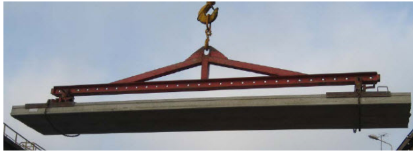
Figure 3.4 - Hoisting of hollow core slabs
