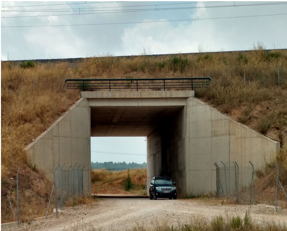
Figure 1.1 – Concrete frame bridge of the Spanish railway network
