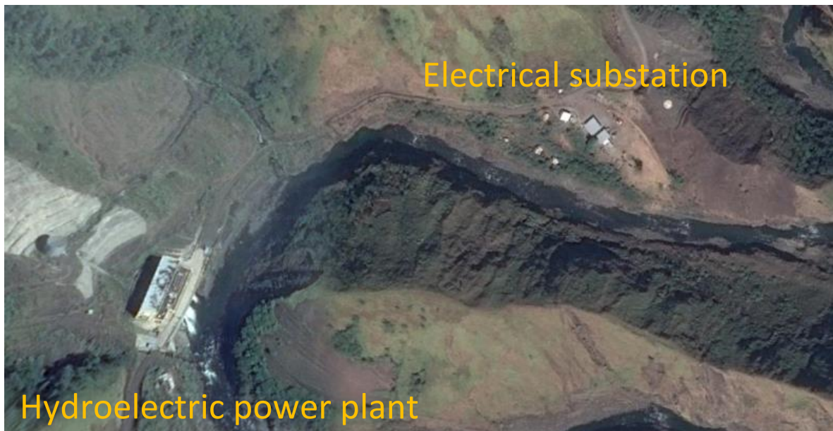
Figure 1. Hydroelectric power plant and associated electrical substation. Image obtained from google earth.
