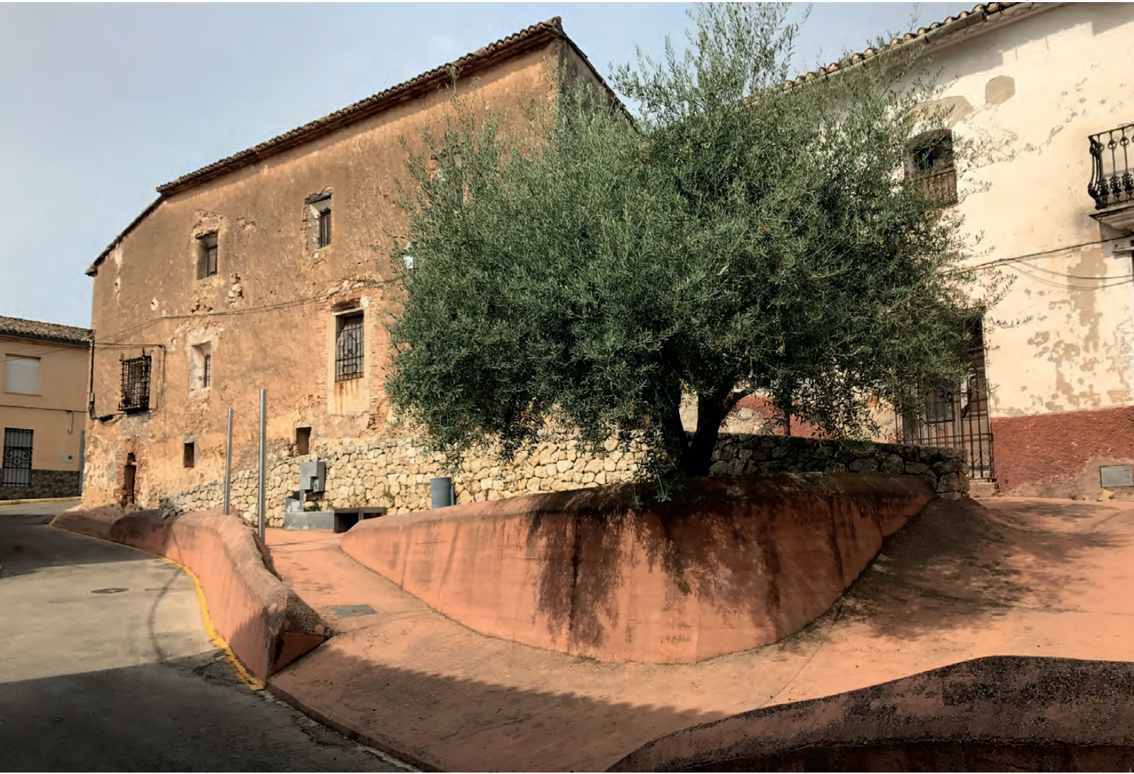
Figura 1. Vista desde la calle inferior (2017) / Figure 1. View from lower street (2017).
