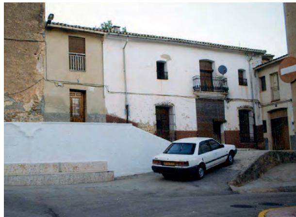
Figura 3. Estado original (1999) / Figure 3. General view before work started (1999).
